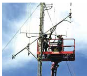
"Cherry picker" at work replacing and adjusting aerial components on the tower.
