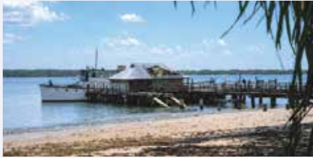
The Bribie Jetty after the cyclone
