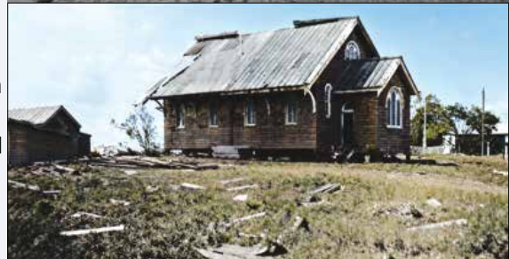
The old Methodist Church that was in Banyra Street, Bongaree, showing damage following The Great Cyclone.
